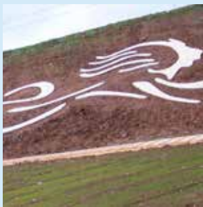
Gateway feature during construction
